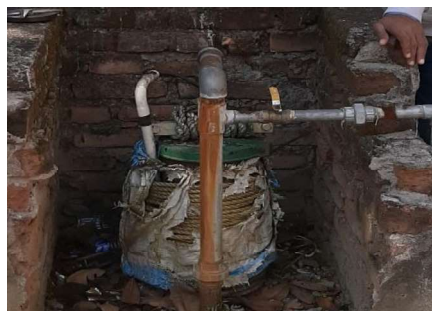
Bore well at Chanch Village
